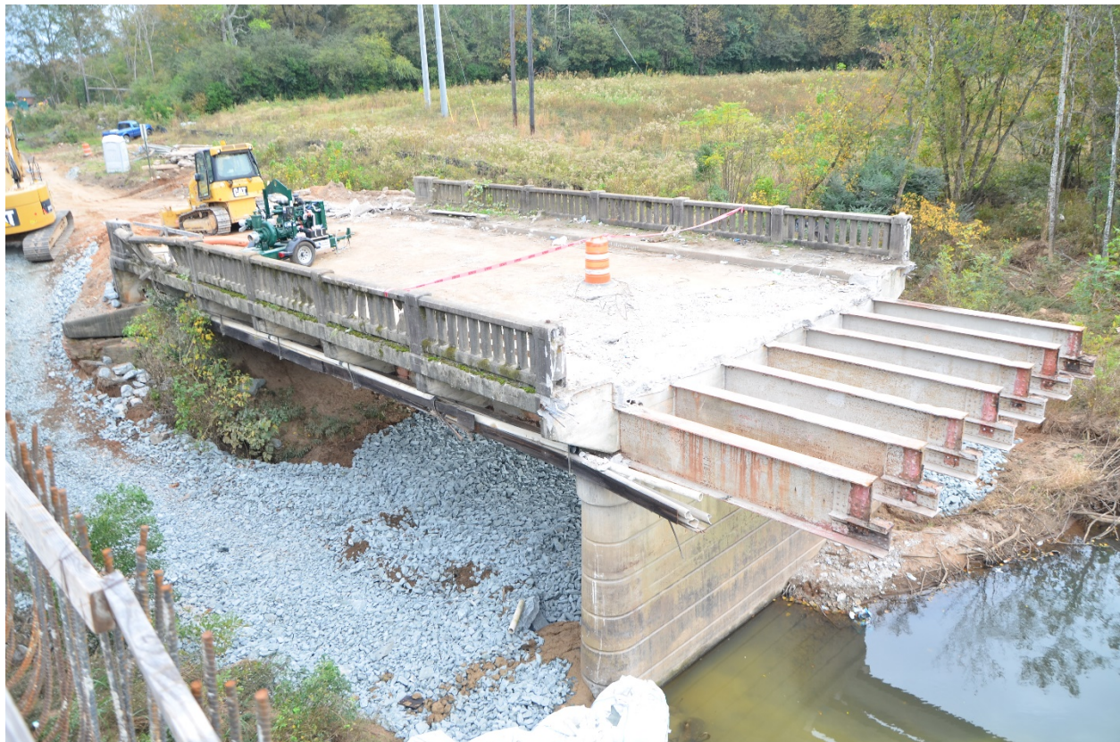
Jeffersonville Road Phase 1 Construction
