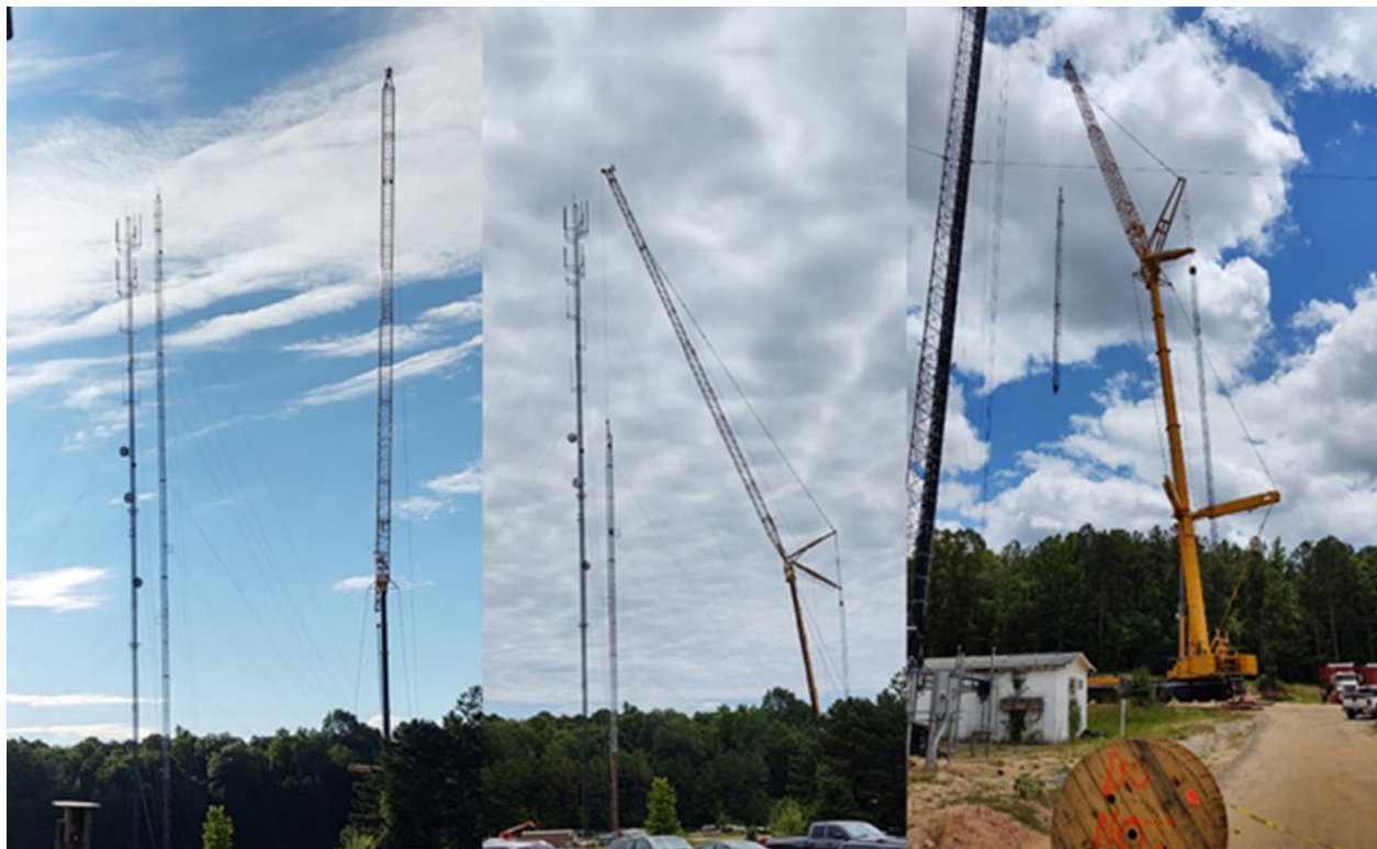
Call Center Motorola Radio Frame Removal
